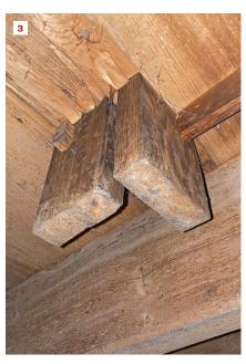
The newel gets a lot of action these days but remains immovable (1). The integral block (2) at the base (about  $6\frac{1}{2}$  inches square) has two tenons cut on its bottom end that project through the floor and are drawn tight to the subfloor by wedges driven into slots in the tenons (3).
