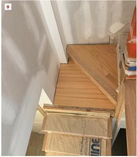
The stair structure ties in with closets at left and right (8)—essential to the client's demands. Here, you can see from above the two winder treads (9)—the lower one is the landing, with the second winder tread on top of it. By code, the smallest dimension of a winder tread must be 6 inches at the handrail line (with a newel or balusters acting as a guard to keep someone from stepping on a tread area less than this) and 10 inches at the walk line 12 inches away.
