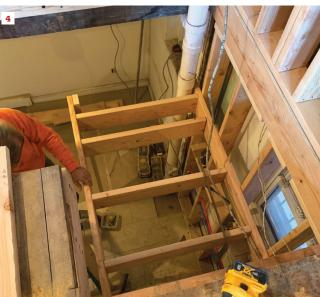
With the new stair opening defined, the exterior wall was furred out to accommodate the water and heating service lines. This required burying an existing basement window that faced a narrow alley (3). The first step in building the rough carriage was to frame the landing, which would become the first winder (4).
