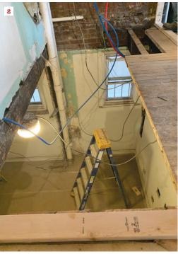
At the outset of the job, the crew began demolition around a plumbing chase, where waste, water. and heat piping would have to be rerouted around the new stair opening (1). As the subfloor was removed, the crew discovered a box-out in the floor from the original straight run of stairs. To make a legal stair, however, they would have to widen and lengthen the floor opening, as well as turn the corner to create an L-shaped opening for a winder (2).
