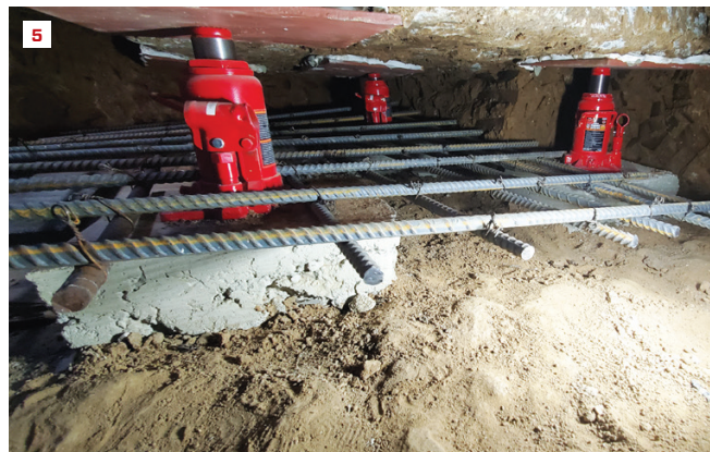
Moment frame. One of the two concrete pillars supporting a Z-shaped lintel (2). Column layout for the new moment frame, south corner (3). A crew member begins work accessing the existing north footing (4). “Sacrificial” bottle jacks are used to support the existing footing during footing underpinning (5).
