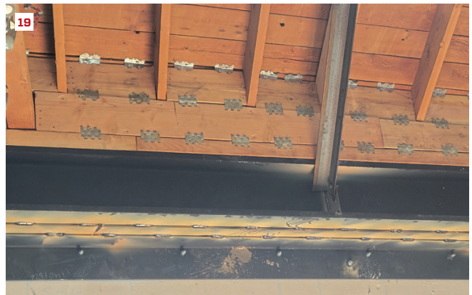
Roof connections. Completed structural work at the angled, wall-to-wall storefront opening includes the steel angle lintel, steel angle diagonal bracing, 2-by blocking, and metal connectors (18, 19).
