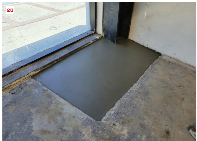
Moment frame. A second concrete pour buries the column base plates and is troweled smooth (20).
