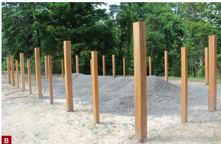
Figure 4. Alternating 6x6 and 4x4 cedar posts were installed in the garden area; here, they have been aligned, plumbed, and braced, and are ready for concrete (A). In this area, the fence design required taller, 6x6 cedar posts with three stainless steel cables run between them at the top to prevent deer from bounding into the garden (B).
