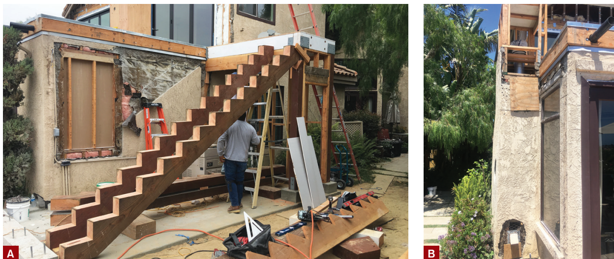
Figure 3. To seismically reinforce the stairs, workers connected a grade beam at the lower landing to the moment-framed upper landing with stringers cut from 4x14 treated Douglas fir beams (A). The chimney was reconfigured to make room for a new direct-vent gas fireplace for the rooftop deck and reframed as a low privacy wall (B).
