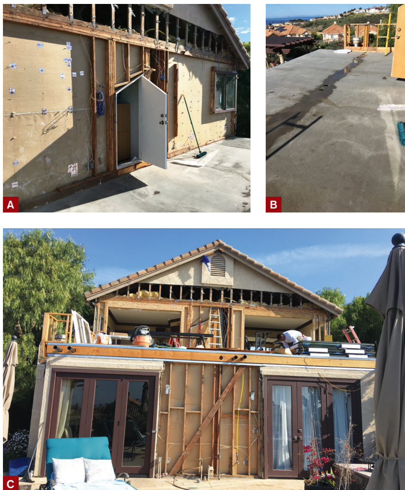
Figure 2. The roof deck was finished with a three-coat stucco finish over diamond lath stapled to the sheathing, followed by a Silcor liquid-applied waterproofing membrane system (A). Water drains through three pairs of roof drains oriented along the centerline of the deck (B). Once the new deck was watertight, workers reframed the wall to install two new bi-fold doors to match the doors on the first floor (C).
