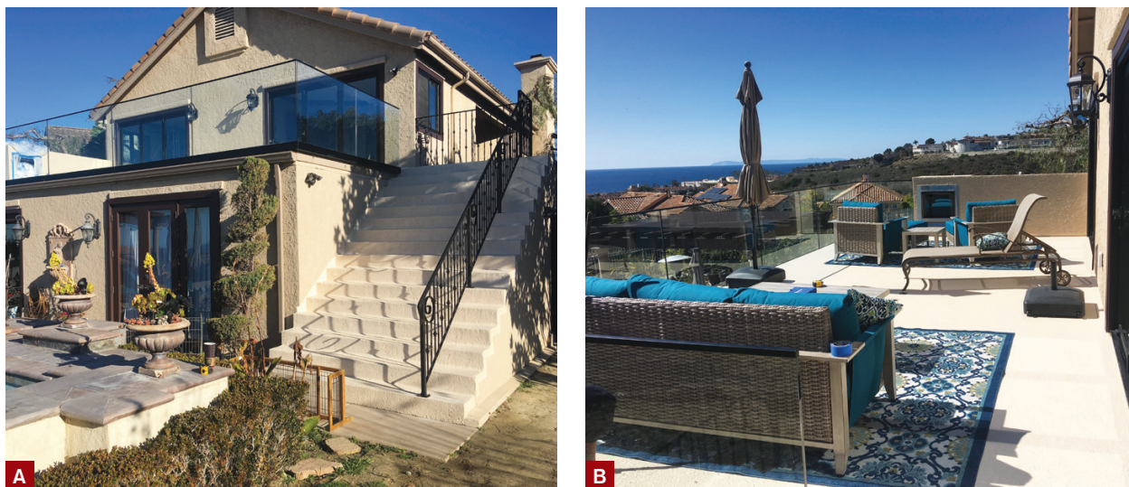
Figure 4. The stairs received the same stucco and Silcor finish as the roof deck, followed by a fire-retardant paint, creating a dry, nonflammable space for storage underneath (A). The stairs were fitted with a wrought iron railing, while the deck's custom-fabricated glass-panel guard system preserves the views of the Pacific Ocean (B).
