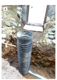
Excavation begins at the basement walkout (1). A length of 15-inch-diameter HDPE culvert installed vertically acts as a catch basin; 4-inch SDR-35 pipe inserted into the culvert's base serves as an outlet (2).
