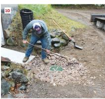
After the HDPE pipe is trimmed closer to grade, the basin's heavy-duty HDPE grate is dryfit to prevent dirt and stone from entering the basin (6) during backfilling (7). The pipe is cut to its finished height, a few inches below slab height (8), and clay soils are used to create a slope away from the house toward the basin (9). Ditch stone is applied around the finished basin (10).
