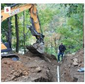
The 75-foot run to daylight is excavated in two sections: first, the walkout end, then the daylight end (3). A crew member joins lengths of SDR-35 with PVC cement (4). The daylight-side piping is complete and ready for backfilling (5).
