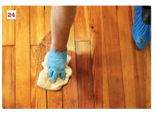
Buffing uses less oil, but the red pad will pick up some excess, mostly at the edges (22). The pad will need to be flipped or replaced as it becomes more difficult to manage. When the pad is removed from the floor, the excess that's left under the pad (23) must be cleaned up immediately (24) before it hardens.
