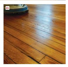
Once the perimeter is cut in, the author fills the center of a red pad with enough oil for a manageable section (17). He spreads the oil quickly in a figure 8 to smear it on the surface (18), and then methodically works it into the field (19) and blends this area with the perimeter (20). Compared to troweling, buffing the oil on creates the least "spitting" (21).
