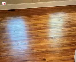
The final step is to polish the floor with a white pad (25, 26). The author feels buffing with pads is the cleanest and most efficient method of applying the oil. However, there is potential for not getting enough oil on the floor, so you need an experienced eye and patient hand to make sure the wood is reaching saturation.
