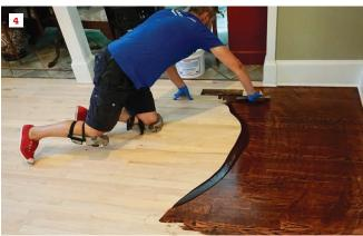
Troweling method. Mike Somodean, a floor refinishing contractor based in Roswell, Ga., shows both sides (1, 2) of the flexible trowel he uses to apply hardening oil. He begins by pouring out a puddle of Ciranova oil, spreading it quickly in a broad sweep and working it skillfully to the edges (3). Working a section as wide as his arm can sweep (4), he covers the length of the room (about 18 feet) in about two minutes.
