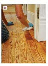
Buffing method. Everything needed by the author for applying hardening oil is shown here (11). A fresh can of Pallmann Magic Oil has room for the hardener so it can be mixed in the can (12). Some of the mix goes into a plastic squeeze bottle to be applied precisely (13). The author immediately rubs it in by hand with a pie-shaped piece of red pad (14). He cuts it in neatly to the baseboard, working a swathe about 6 inches wide around the perimeter of the room (15, 16).
