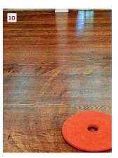
After 10 to 15 minutes of "dwell" time, a crew member comes in behind Mike to further work the oil into the wood with a buffer fitted with a red buffing pad (5). When the wood reaches saturation, excess oil will "spit" out (6). He changes the red pad out for a white one (7) to absorb the residue (8) and polish the floor (9). The crew works the floor in sections to stay ahead of the oil before it hardens (10).
