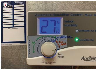
Cartridge steam humidifiers emit steam into HVAC ductwork when called for by the humidistat (1). In the author's climate, his company recommends clients set controls at 35% RH or lower (shown here marked up with colored pens), based on its experience that most buildings can handle 40% to 45% relative humidity in winter without moisture problems, and allowing for some inaccuracy or drift in the sensor (2).
