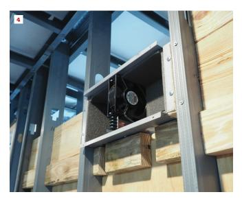
Wall emitter boxes are used with steam cartridge units where ductwork is not available to distribute the humidity (4). Humid supply air is hosed from a steam cartridge unit, typically housed in a nearby mechanical room or closet (5), to the emitter box, which has a built-in fan to mix air with the steam. Grills can be a bit obtrusive unless hidden in a hallway or other less visible location (6, 7).
