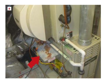
Pad humidifiers often drip or splash a bit of water, as on this galvanized metal pan, which has seen enough water to start rusting (8). Steam humidifiers put out a tremendous amount of moisture, and if the HVAC fan doesn't circulate it throughout the house, it will turn into water in the ductwork and leak, as seen in the two photos at right (9, 10). The author's company now uses a secondary safety device to ensure the fan is operating before the humidifier will run.
