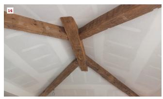
Once they were satisfied with the fit of the first hip beam, workers fastened it in place using long trim screws for the wood-to-wood connection to the ridge beam (11) and structural screws for the connection to the house framing (12). After honing their technique on the first hip beam, they were able to install the remaining three beams quickly (13), and the ceiling was soon ready for the paint crew (14). When viewed from floor level, the screw heads are virtually invisible.
