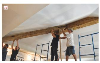
The crew cut the ridge beam long by 2 inches to allow for fine-tuning the fit, then lifted and propped it in place (5) to scribe both ends for the final precise fit (6). Before installation, a worker drilled a hole in the middle of the beam for an electrical fixture (7). The crew fastened the beam to the framing above with long structural screws (8, 9). The first hip beam was cut long by 3 inches, then gradually trimmed to fit following the same procedure as for the ridge beam (10).
