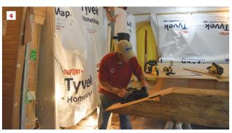
After determining the angle where the sloped and flat sections of the ceiling converged, the author made an MDF template and used it to mark that angle on both sides of the beam (1). Next, he cut to the lines with a circular saw at maximum depth (2) and finished the cut with a chain saw (3) while a helper supported the offcut. Finally, he smoothed out the cut with a handheld power planer (4).
