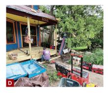
After shoring up the porch roof with temporary supports (A), workers removed the old porch. In addition to inadequate footings, the porch's roof system had been simply toenailed to the wall sheathing and was pulling away (B). After digging and pouring new footings (C), the crew installed new porch framing, with the joists oriented parallel to the house (D).
