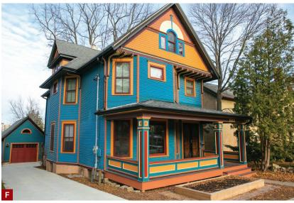
The crew installed blocking around the new pressure treated posts supporting the roof, then reinstalled the porch's original columns and colorful balustrade (E). The project included a new garage, designed and finished to fit with the character of the house (F).
