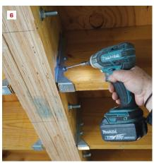
Overcut joists. Gaps at joists ranged from 1/4 to 1/2 inch wide (1). Repair work began with drilling for 1/2-inch threaded rod on 16-inch centers (2). Ernesto and Toby Bonilla of Great Lake Builders worked together to tighten the nuts, drawing the beam plies together (3). All the undersized nails had to be pulled from the joist hangers (4, 5) and replaced with structural screws (6).
