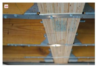
**Tight quarters.** Every hole had to be filled with a fastener—a feat that can be challenging in narrow bays. Here Toby used an angle drive (7) to get the job done (8). Tension ties. Ernesto screwed off 20-gauge steel straps to the bottom edge of the joists (9). Each pair of joists abutting the LVL beam was tied together with these straps (10).
