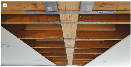
Compression blocks. Toby nailed off 18-inch-long 2x6 blocks at the top edge of the joists (11). These blocks hit the joist hangers and screws, so the crew eased the corners (12) and in places used shims (13) to get a tight wood-to-wood connection. The result of all the repairs (14) is a single assembly rather than a collection of disconnected parts.
