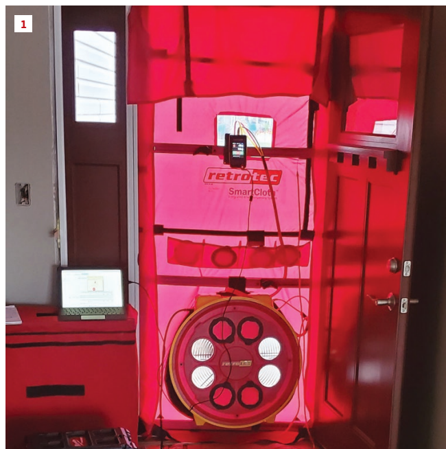
Blower door testing a home requires much more than simply setting up the equipment and running it.
