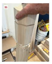
Six inches of old post projects above the main sleeve, enough to glue on the cap piece (30, 31), which is pinned plumb and stable using trim-head screws before the glue sets.
