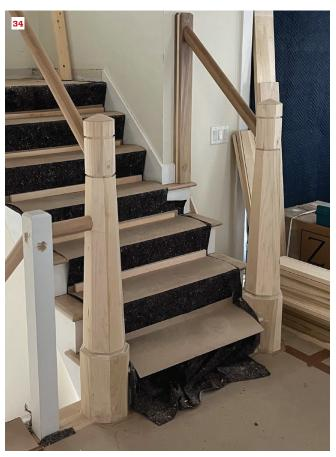
The oversized handrail had to be let in to the post. The author made a router jig and used a bearing-over straight router bit to make the recess (32). A slightly oversized recess accommodated the angled insertion, later filled with two-part epoxy wood filler and sanded to a seamless fit (33). The retrofit glued-in bases provide a stiff newel-rail assembly (34).
