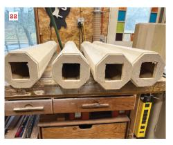
To align sleeve components around the existing 4x4 post, U-shaped plywood is glued together to form a 4x4 cutout (20), the corners chamfered and fine-tuned on a sander (21) to fit inside post and base ends (22).
