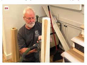
The base is cut out to drop onto the floor (27). After the author scribe-tunes the fit, he glues the base in place with heavy-duty construction adhesive (28). Squeeze-out is cut away after curing. To fit the post inside the tapered sleeves, the author power-planes the old post corners until the sleeves drop into place without resistance (29).
