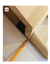
The base section, fitted over the old post, is plumbed (23) and traced onto the existing starter tread (24), to be let in. The outline is cut from the tread (25), and the riser lines traced onto the base (viewed looking up under the starter tread) (26).
