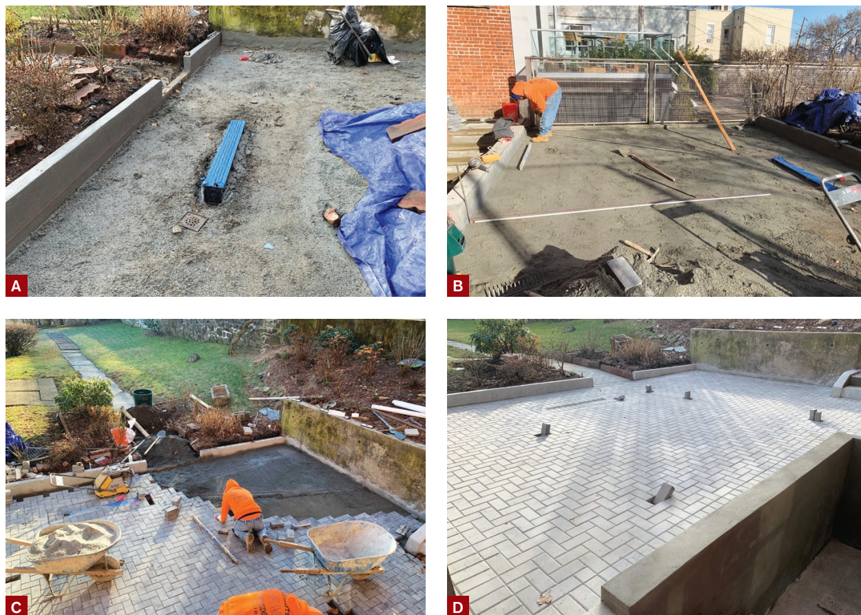
Figure 2. A new linear drain was installed to improve drainage (A), along with a properly sloped QP (quarry process) setting bed for the new concrete patio (B). These measures were needed to capture water draining from the narrow backyard, which is at a higher elevation (C). Upturned pavers mark the locations of the new deck footings (D).
