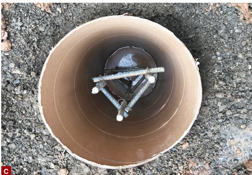
Figure 1. Workers dismantled the existing steel deck and concrete patio pads (A) and replaced an entry door (B). The six new poured-concrete deck footings were reinforced with triangular rebar cages (C).
