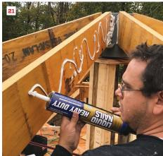
The hip rafters are connected to the steel circular ridge with structural screws driven up through holes in the ridge into each rafter (20). Construction adhesive and structural screws were used to join the double-LVL hip rafters together (21). At the ridge, metal straps reinforce the connection between opposing rafters, while custom-fabricated brackets connect the hip rafters to the plates (22). Then the crew installed common rafters, subfascia, and roof sheathing (23).
