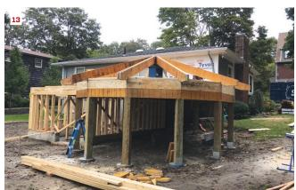
The dodecagon's 12 double-LVL hip rafters hang from a customfabricated circular steel ridge (10). Working off the level floor deck made it easier to lay out the rafters (11). The plumb cuts where the rafters meet the ridge needed to be notched (12) to allow the rafters to fit over the connecting flanges at the ridge (13).
