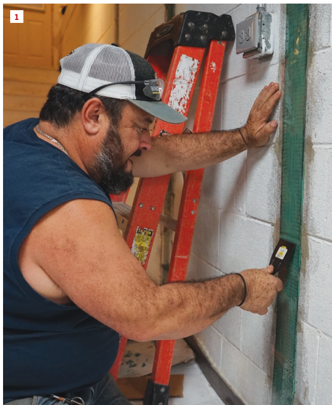
Toby Bonilla of Great Lakes Builders smooths out the two-part epoxy used to reinforce a block foundation wall.
