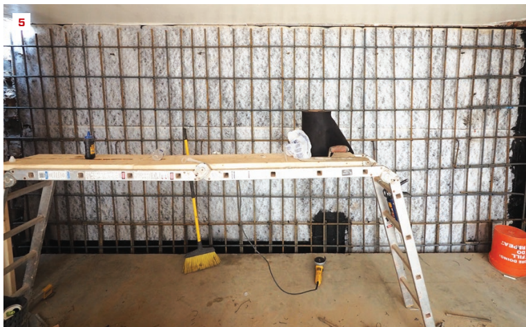
At the slab-to-wall juncture, the existing slab was saw-cut in order to lock in the bottom of the new heavily-reinforced concrete "liner" wall (4). The cut edge also allows room to drain the wet side of the drain board to daylight via two sub-slab PVC drainpipes (see section illustration, facing page).
