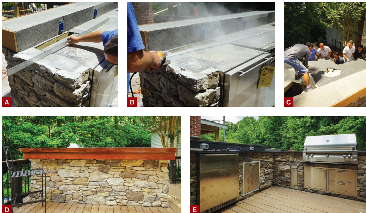
Figure 4. Workers checked the top of the cabinet surface with straightedges (A) and used a grinder to remove high spots (B) to make sure it was flat prior to installing the granite countertop (C). Ipe trim on the bar overhang (D) offers a warm contrast to the stone veneer cladding (E).
