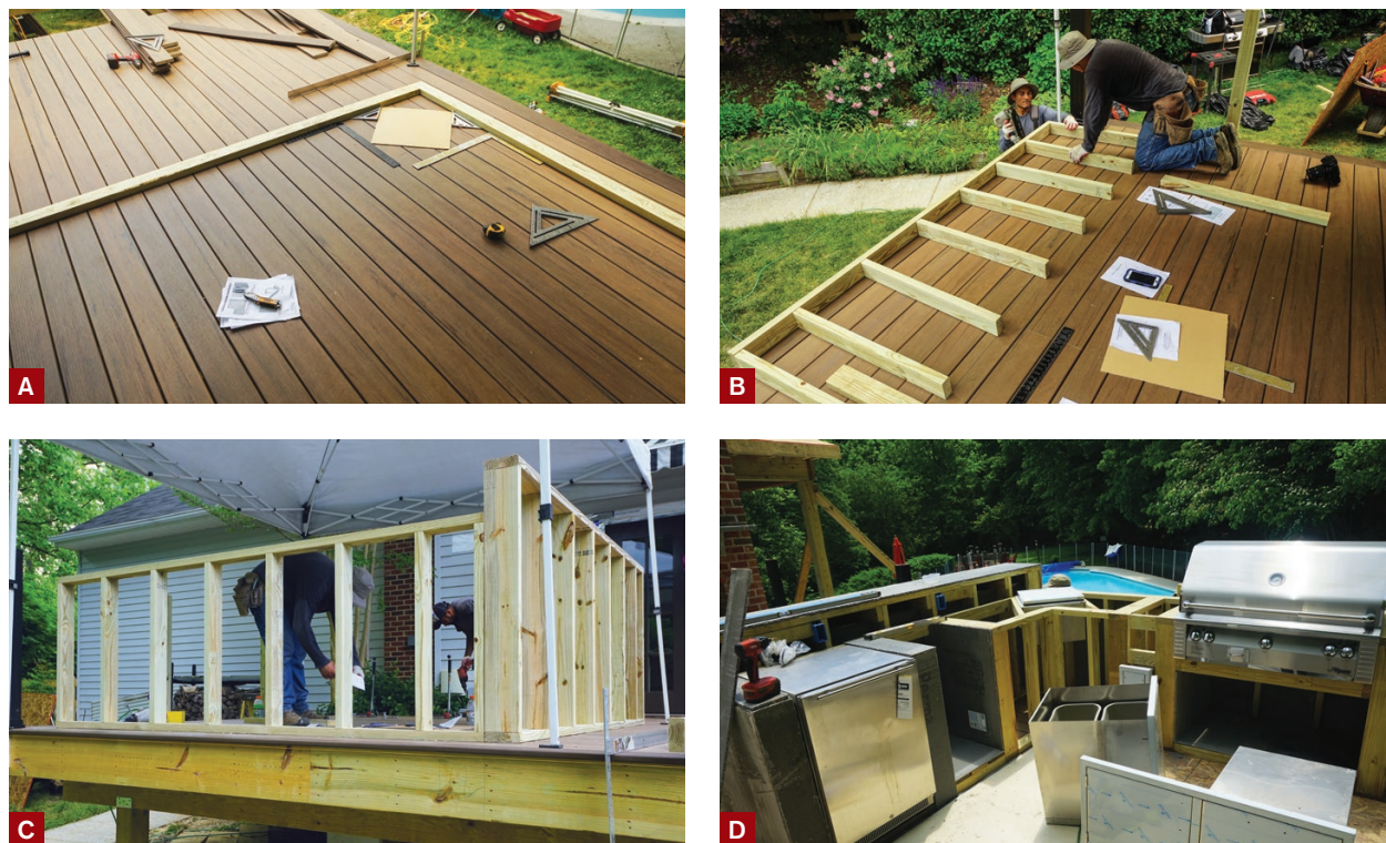
Figure 2. Using cardboard templates sized to fit the appliances (A), workers framed the kitchen's perimeter walls on the deck (B) with pressure-treated 2x4s and 2x6s, then screwed them together and through the decking into blocking installed between the joists (C). The cabinet walls are clad with cement board over a vapor retarder (D).
