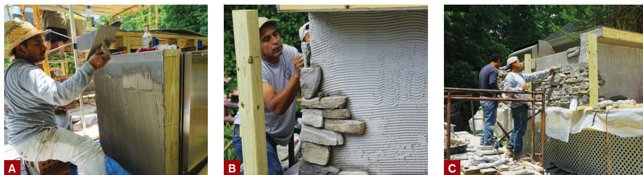
Figure 3. Masons troweled on a mortar scratch coat over galvanized diamond lath fastened to the cement board (A), then allowed the mortar to cure overnight. When applying the manufactured stone veneer, they started at the corners (B) and worked in sections (C), back-buttering each stone and pressing it into the scratch coat.
