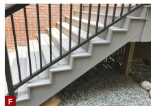
A closed stringer detail looks good but can trap debris (A). On open-stringer stairs, the author cuts nosing returns to mimic the look of interior stairs (B, C). The author's "two-tier" style looks good with contrasting treads and risers (D). The "waterfall" style requires more blocking (E) and can be used with contrasting or single-color tread-and-riser combinations (F).
