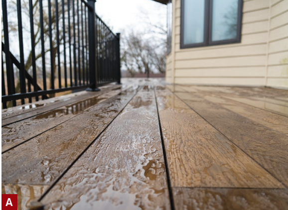
The enhanced grain of Millboard decking offers good slip resistance (A). While bullnose boards are available for stair treads, the author typically uses standard square-edged boards with Fortress's steel stair framing (B).
