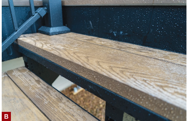
The enhanced grain of Millboard decking offers good slip resistance (A). While bullnose boards are available for stair treads, the author typically uses standard square-edged boards with Fortress's steel stair framing (B).
