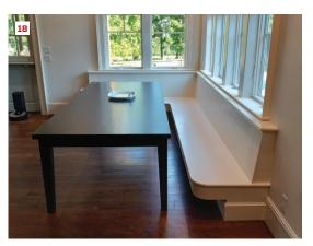
For the corners, the author used his patterncutting technique to make multiple identically curved pieces to glue into radiused blocks (15). Dominos join the two parts of the bench seat together where they meet at right angles (16, 17). The bench seat was given a paint finish to match the rest of the room's interior trim (18).
