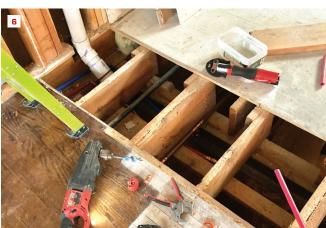
tougher install because he had no play to work the PVC into position. This worked all the way to the last joist, which was only  $4\,^1\!/2$  inches away from the rim joist, where the hole had to drop below the middle third. Structurally, this was not a huge concern, because of the close spacing, but Joe still installed the required glued plywood reinforcement to the joist before drilling the hole and running the drain.
