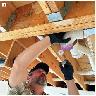
Relocating the drain lines to the exterior walls proved to be challenging: To preserve the integrity of the joists, the holes needed to be within the middle third of each joist, but they still needed to drop to provide drainage. To succeed, Joe had to drill his holes to the exact outside diameter of the pipe, leaving very tight tolerances for running the pipe straight through (1). The old ABS lines were replaced with PVC (2) everywhere except where vent stacks tied in.
