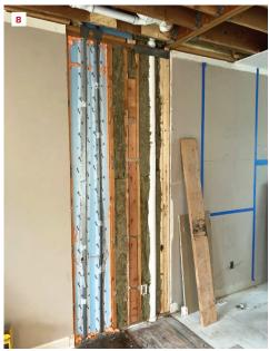
To protect the new supply runs, the author used half of a metal-framing track to create an angled piece of steel. Short pieces of PEX cushion an electric line that runs behind the pipes (7) before the steel angles are taped in place against the foam (8) and the surrounding walls are insulated, ready for drywall.
