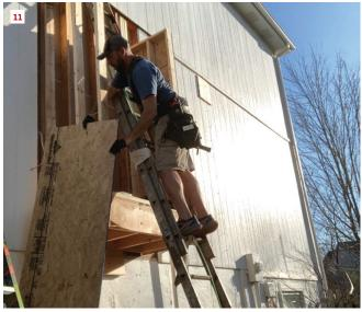
**Fireplace bump-out.** While Joe was busy with the plumbing, followed by the relocation of the gas piping, I turned my attention to framing a bump-out on the exterior wall to accommodate the new fireplace.
