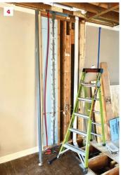
New supply lines tied into the existing copper with press fittings (3). Note the ABS vent connection using Fernco fittings with rubber sleeves and hose clamps. Before running new supply lines in the exterior wall, the author insulated the bay with rigid foam (4). A press tool was essential for joining new PEX to existing copper in tight framing bays (5, 6).
