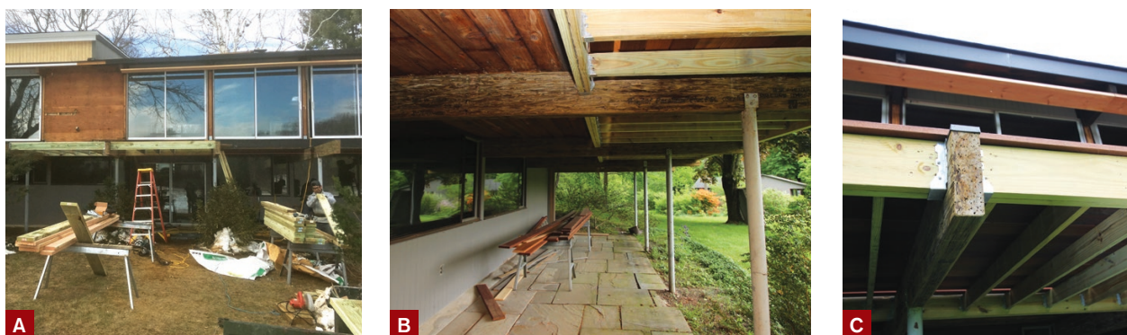
Figure 4. The cantilevered main-level floor and replacement deck are supported by seven 4x12 parallams, then flush-framed with 2-by pressure-treated stock (matching the previous deck's framing layout) (A, B). The existing steel columns were reused to support the ends of the parallams, while the new beams were cap-flashed to prevent rotting (C).
