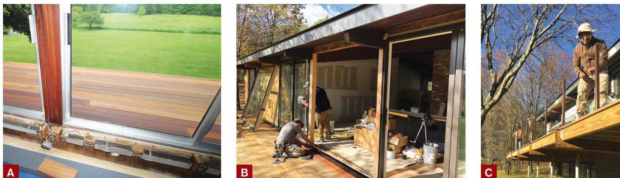
Figure 5. At the sliding doors, workers removed the 8-inch-high rise that accommodated hydronic baseboard (A) and replaced the three existing sliders with two Marvin Ultimate sliding patio doors flanking a fixed glazed center panel (B). Crew members installed a stainless steel cable-railing system (C), shown here before the ipe top rail was installed.
