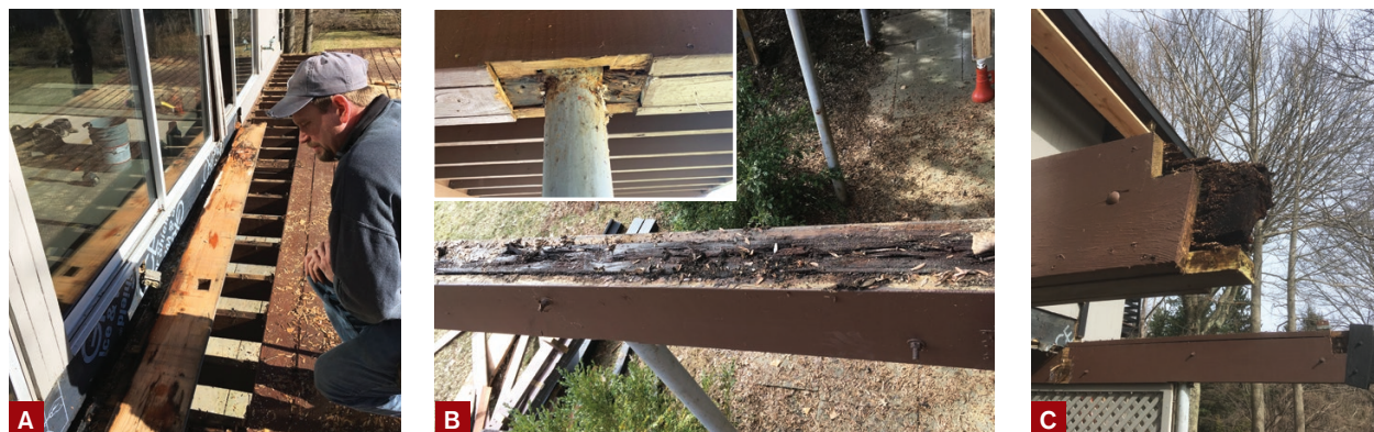
Figure 1. While removing the existing decking (A), crew members discovered the home's original 4x12 fir beams were encased in pressure-treated stock, not flashed, and severely deteriorated (B, C). The steel column connections that helped support the cantilevered ends of the beams had sunk into the rotted Douglas fir (B, inset).
