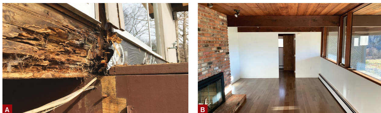
Figure 2. Years of water infiltration had damaged the raised thresholds under the sliding doors (A). From the interior, the 4x12 fir beams that span the width of the home look intact (B), and it was assumed (wrongly) that the 14-foot "cantilevered" lengths of fir (which supported the cantilevered floor and original deck) had been removed when the original deck was replaced.
