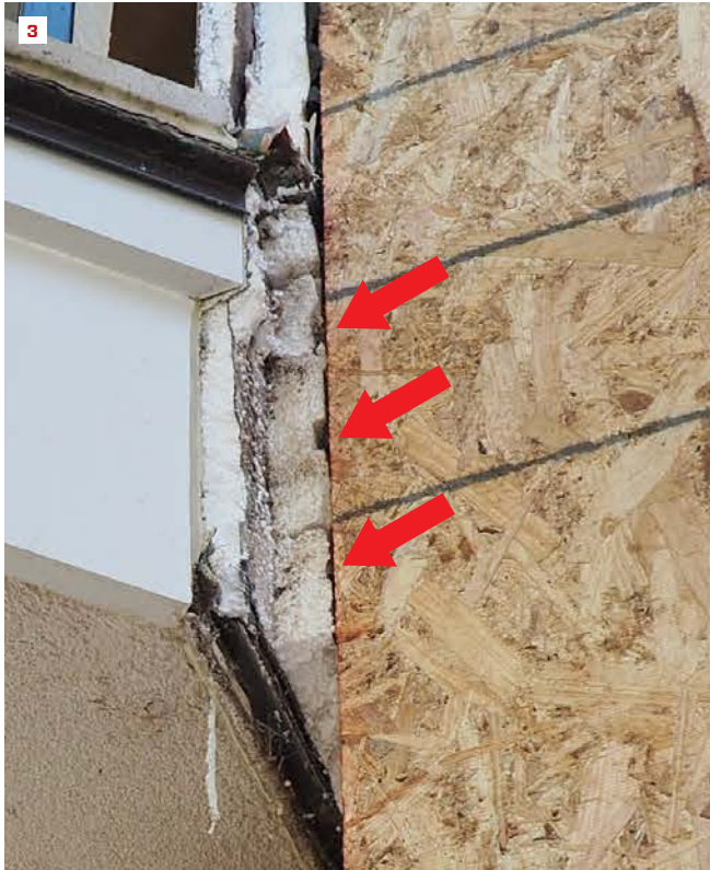
Drainage channels (arrows) were installed horizontally at the band-joint area on this house, blocking the vertical channels above (3). (We had already replaced the sheathing visible here, since the trapped water had rotted out the original OSB.)
