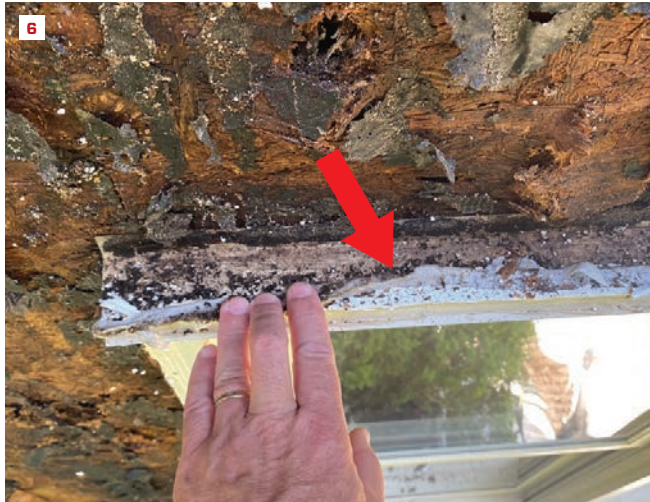
The heavy bead of sealant on top of this window head flashing blocked the drain path from the vertical channels above the window (arrow) (6) .
