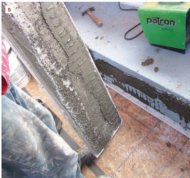
Drainage channels (arrows) were installed horizontally at the band-joint area on this house, blocking the vertical channels above (3). (We had already replaced the sheathing visible here, since the trapped water had rotted out the original OSB.)
