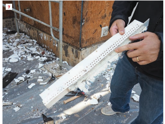
Heavy caulking blocked the weep holes in this plastic track installed at the bottom of the drained EIFS on the wood walls (7) . The trapped water caused water staining all along the bottom of the wall, visible in the background.
