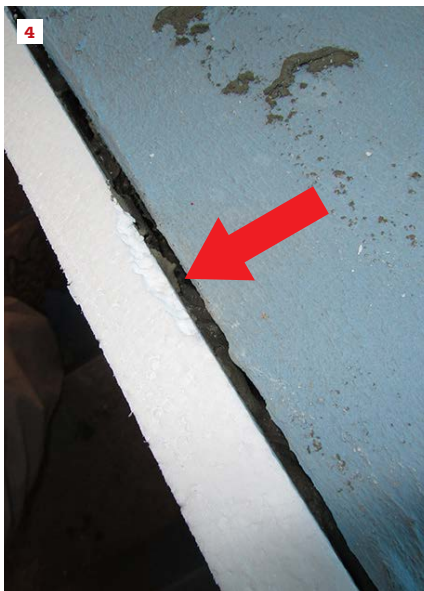
Drainage channels (arrows) were installed horizontally at the band-joint area on this house, blocking the vertical channels above (3). (We had already replaced the sheathing visible here, since the trapped water had rotted out the original OSB.)
