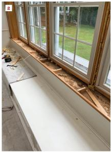
The clad windows in the existing box bay were in good condition, but there were signs of water damage to the trim on the exterior (1). More signs of water stains and rot were visible on the subsill once the stool was removed (2).
