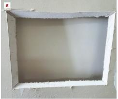
To repair an existing hole, cut out the patch first, place it over the hole, and trace its outline (7). Cut to the line with the blade at a 30- to 45-degree angle (8), then bevel the edges of the patch to the same angle (9). Fine-tune the fit by pressing the patch into the opening and shaving off high spots with the blade fitted between the patch and the cutout (10). A few drywall screws will help hold the patch in place while the mud dries (11).
