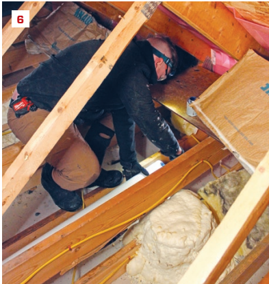
A crew member replaces a length of 4-inch flex duct run from a bath fan with 4-inch rigid PVC piping. The PVC duct sloped \frac{1}{4} inch per foot toward the soffit vent. In the foreground, a recessed light is air-sealed with a site-built OSB cover foamed in place (6).
