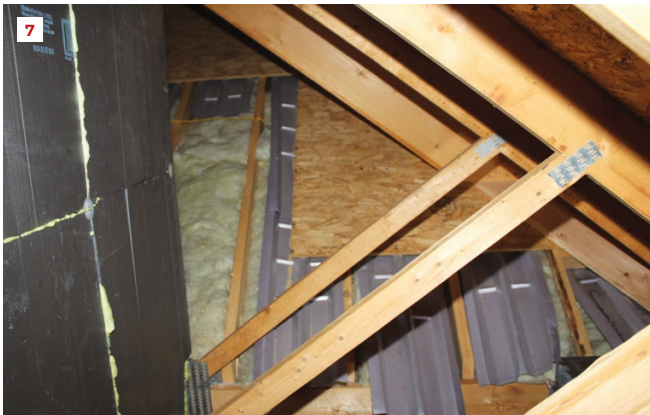
Note the existing ineffective thermal control where the garage wing intersects with the main roof, with large areas of exposed fiberglass and loosely placed Propavents (7).
