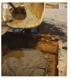
With the shoring in place, the crew cuts open the basement slab (5) to dig 36-by-36-by-18-inch footings for columns to support the new steel I-beam. Note the chairs (6)—called "bolsters" in the Midwest—to keep the rebar elevated when the footing is poured (7).
