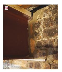
Prying against a joist (16, 17) pushes the first beam section into the pocket. Grouted into the wall after the columns were set, the beam bears on a steel plate (18). Note the top plate on the beam installed with powder-actuated fasteners prior to lifting.
