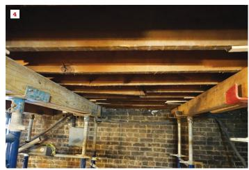
A partition wall, which sits directly above these damaged first-floor joists, was not designed to bear the added loads imposed by an underbuilt roof (1-3). To begin repairs, the crew erected emergency shoring (4) on each side of where a steel beam will be placed to support the loads.
