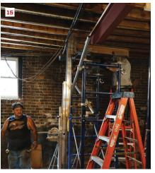
Because space was limited, the new steel beam had to be lifted in two sections, using a Sumner material lift (14). With the lift holding the first section in place, shoring is erected below the beam (15). At this stage, the beam is slightly low to allow the crew to move it laterally into a beam pocket in the far wall of the basement.
