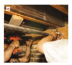
Toby Bonilla grinds down the high spots on the basement wall in preparation for installing an LVL ledger (8). The ledger is secured with threaded rod epoxied into the wall (9, 10).
