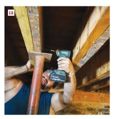
Working together, Toby and Ernesto Bonilla sister new LVLS to the existing joists (11). With one end of the LVL sister bearing on a beam or ledger, the opposite end is jacked up to align with the bottom of the existing joist (12) and secured with structural screws (13).
