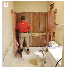
Before installing backer board, the author checked the wall framing (6) and planed any bowed studs so that the wall would be flat (7). Clips hold the shower base in place (8). A new bench seat will be installed in the gap between the shower base and the wall (9).
