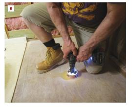
After removing the existing fiberglass tub (1), the author cut back drywall and installed blocking for new grab bars (2). Using the new shower base as a pattern (3), he marked where the flooring and underlayment needed to be cut back (4) and where a hole for the shower drain needed to be drilled (5).
