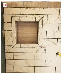
The author coated the tile backer board with a liquid-applied waterproofing membrane (14), then installed 4-inch-by-12-inch tile in a subway pattern (15). Tile colors were chosen for high visibility (16), while the new grab bars make all areas of the 5-foot-wide bathroom safer and more accessible (17).
