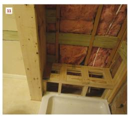
To make the short, <sup>3</sup>/4-height wall that partially encloses the shower bench, the author framed it with 2x6s tied with plenty of blocking to the existing framing (10), and covered both sides with <sup>5</sup>/8-inch plywood (11). A diverter valve supplies water to either the showerhead (12) or a handheld shower over the bench seat (13).
