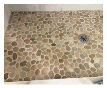
Irregular stone pebbles add a natural design element to a tiled shower but should be installed over a base with more pitch than normal to allow for better drainage.
