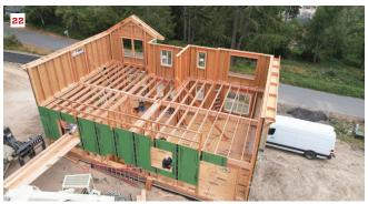
The floor system is hung from ledger boards that are fastened to the wall framing with structural screws (19, 20). To help flatten the walls, the author temporarily screws an I-joist to the studs to pull them into plane while he installs the ledger boards (21). After the floor system is in place, construction can proceed conventionally (22).
