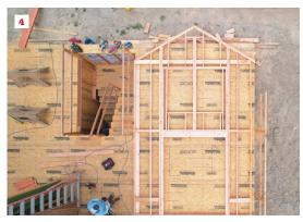
To stiffen a balloon-framed wall for lifting, the author doubles up the 2x6 king studs on either side of openings (1). The 2x6 blocking installed on the flat will support panel edges (2), while solid 4x6s are used for both panel edge support and fire blocking where needed (3). Fully framed from the bottom plate to the gable, this wall is ready for sheathing (4).
