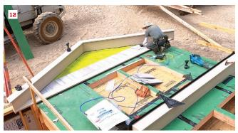
Details such as this bump-out (9) and soffit (10) are easier to build while the wall is flat on the ground. Windows and siding can also be installed before the wall is lifted into position (11), as well as gable rake trim (12).
