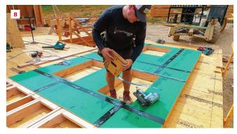
Sheathing is installed from the top plate down, leaving the framing exposed at the bottom of the wall (5). The 4x8 panels are aligned vertically and nailed to the framing 6 inches on-center (6). The author uses a router to cut out window and door openings (7). Where required for seismic reinforcement, the author installs continuous strapping above and below openings (8).
