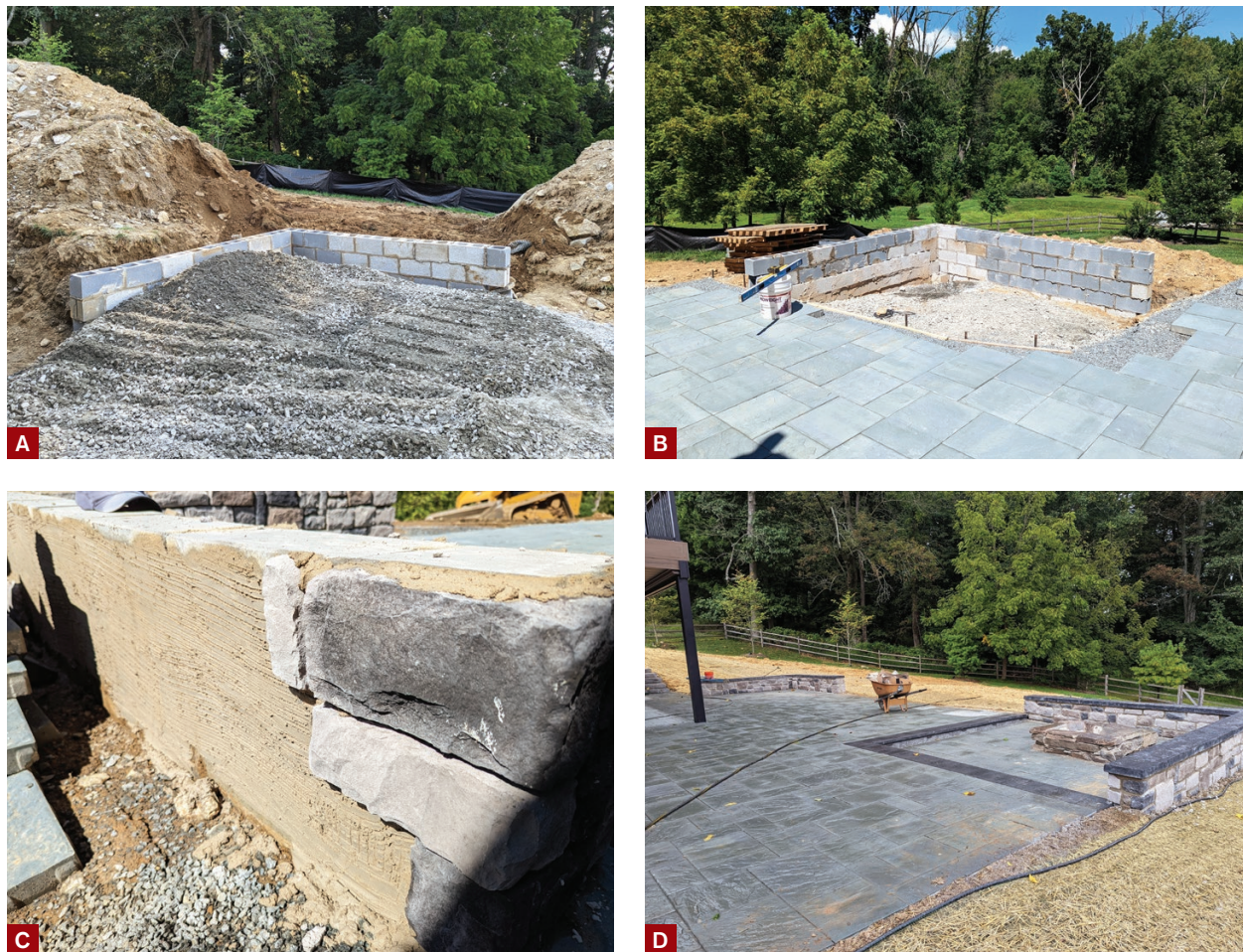
Figure 3. The sitting walls at the corners of the cast-stone-paver patio are supported by full below-frostline footings (A), which prevent heaves and cracks and stabilize the edges of the patio (B). The block walls are finished with manufactured stone veneer (C), and capped with manufactured pavers that match the edging around the sunken fire pit (D).
