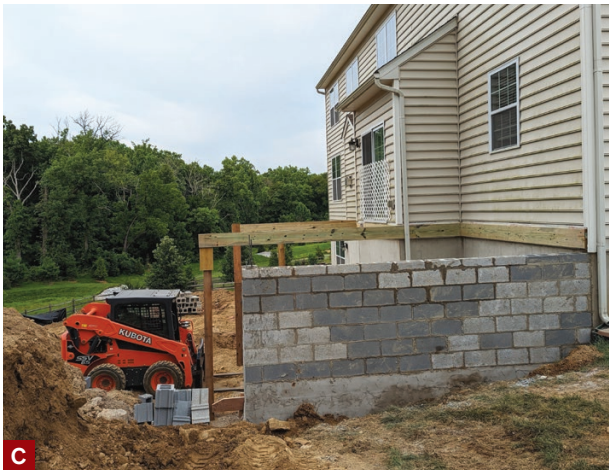
Figure 2. Shown here is the formwork for the footings (A) that support the engineered block retaining wall (B) built to partially enclose a dry storage area underneath the deck. After the retaining wall was built, the author's Kubota SSV65 skid loader was used to lift the heavy deck beam into position (C). The storage room has a concrete slab floor (D).
