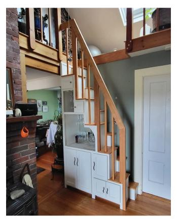
New provisions in the 2024 edition of the IRC allow for sleeping lofts of less than 70 square feet, with access from a ship's ladder or alternating-tread staircase, as shown here.
