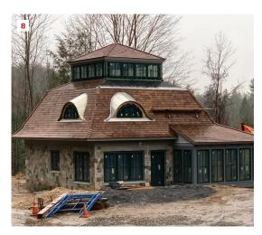
The panels could be laid in place as needed as the crew worked their way up the roof, making them easier to work with than a roll of material that has to be installed in long courses (6). The red-cedar hip cap shingles were custom-fabricated off site to match the specific roof pitch where they would be used (7). Because shingles are fully supported by the rigid panels, they won't flex or crack under a worker's feet as they might with a more compressible, fabric-style rainscreen material (8).
