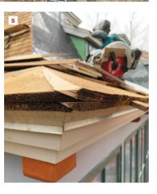
Ventgrid12 plastic rainscreen panels can be used under siding (1) as well as roofing. The roofing crew installed the 4-by-8-foot panels over Grace Ice & Water Shield membrane, which the general contractor had installed (2). Workers used saws and snips to trim panels to fit at hips and around vents (3, 4). The panels are flexible enough to conform to the flared roof deck (5).
