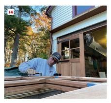
Heavy-duty hinges made by RealCraft (realcraft.com) were used to hang the 150-pound doors. After the hinges were clamped in place (12), holes were drilled for the through-bolts (13), and the hinge strap and back plate were bolted together (14).
