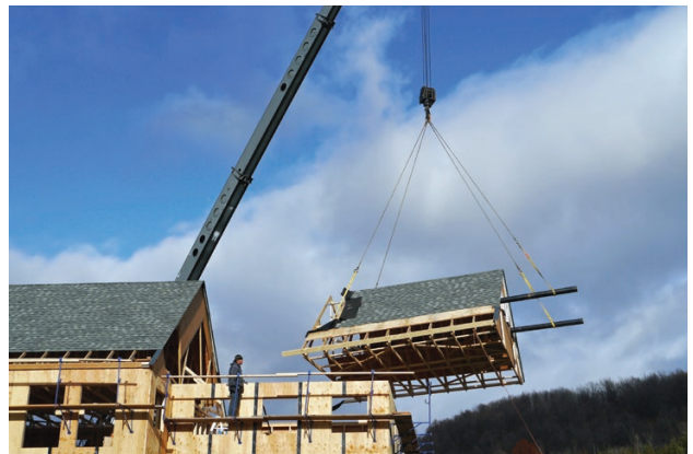
Prefabrication doesn't always need a factory. Lee McGinley found it safer and more efficient to build this roof assembly on the ground and crane it into place.
