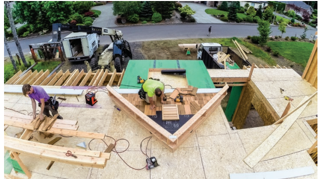
Building faster and safer: Tim Uhler installs the siding, vent, and eaves on rake walls before lifting them in place.
