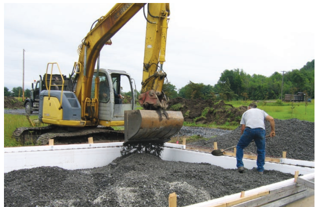
A range of new technologies in residential construction have sped up construction while improving energy efficiency. ICF foundation forms are an example.
