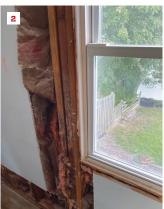
Most of the termite damage to the framing occurred on the ground floor in the living room (1). Damage was also found around a secondfloor window (2), so the author removed the drywall and insulation along the bedroom wall to determine its extent (3). In several structurally significant areas, termites had transformed the wood framing into a papiermâché-like material (4, 5).
