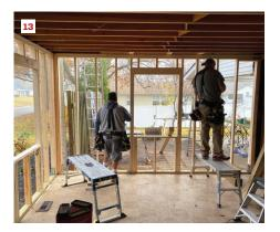
Before reframing the walls, workers installed a copper termite barrier over the edge of the slab foundation (11), then used wedge anchor bolts to fasten new pressure-treated plates to the slab (12). Once the walls had been reframed and fitted with the proper hardware to reinforce the connection to the existing framing and foundation, the post jacks were slowly removed (13).
