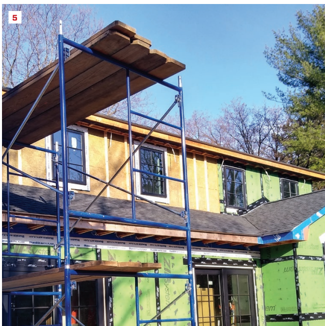
After wrapping the window bucks, the crew installed exterior insulation abutting them.
