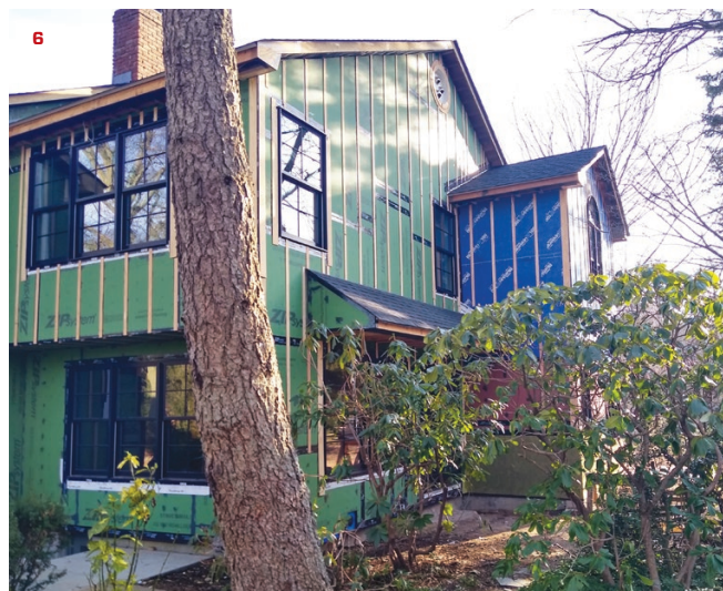
Strips of 1/4-inch marine plywood act as the rainscreen. The windows are open to drain behind the siding and out.
