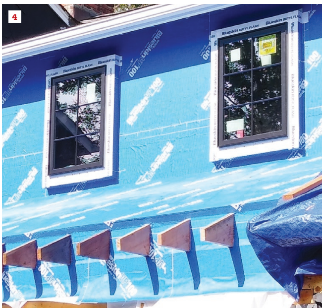
Strips of 1/4-inch marine plywood act as the rainscreen. The windows are open to drain behind the siding and out.
