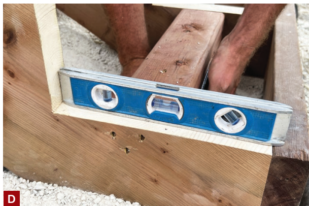
Figure 2. Here, the author is installing double 2-by blocking cut to fit between a pair of stringers (A). After nailing off the stringers to the blocking (B) and nailing the double blocking together (C), he turns the nut underneath the saddle until the stringers are level (D). Then he repeats the process for each pair of stringers until the stair is level from side to side and from front to back.
