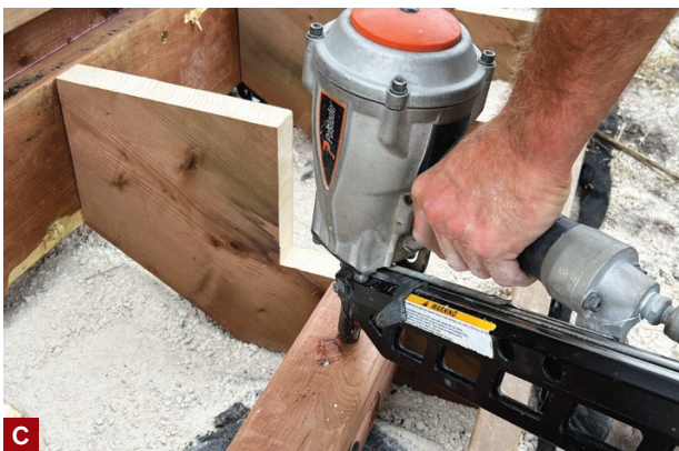
Figure 2. Here, the author is installing double 2-by blocking cut to fit between a pair of stringers (A). After nailing off the stringers to the blocking (B) and nailing the double blocking together (C), he turns the nut underneath the saddle until the stringers are level (D). Then he repeats the process for each pair of stringers until the stair is level from side to side and from front to back.
