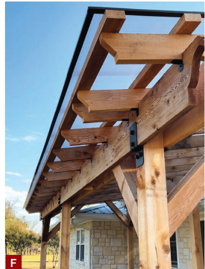
Figure 2. Angle brackets are used to fasten the rafters to the beams, along with structural screws driven down through the tops of the rafters (A). The roof panels are supported by 2x4 purlins and are fastened to them with special metal clips (B). Friction-fit connector caps are tapped into place with a mallet to cover the raised seams between panels and prevent leakage (C), then plugged with matching end caps (D). The ends of the hollow panels are covered with a special vent tape followed by a flute cover, allowing for ventilation while blocking access to insects (E). The outside edge of the last panel is cut to fit, then covered with a metal U-edge profile that is screwed to the purlins (F).
