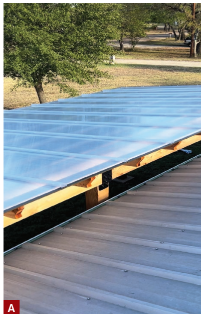
Figure 3. Raising the inner beam of the free-standing pergola above the eaves of the home's hipped roof allows for air circulation as well as the recommended slope (1 inch in 4 feet) for the polycarbonate roof panels (A). The panels chosen for this patio cover allow plenty of natural light into the home while providing shelter from rain and snow (B).
