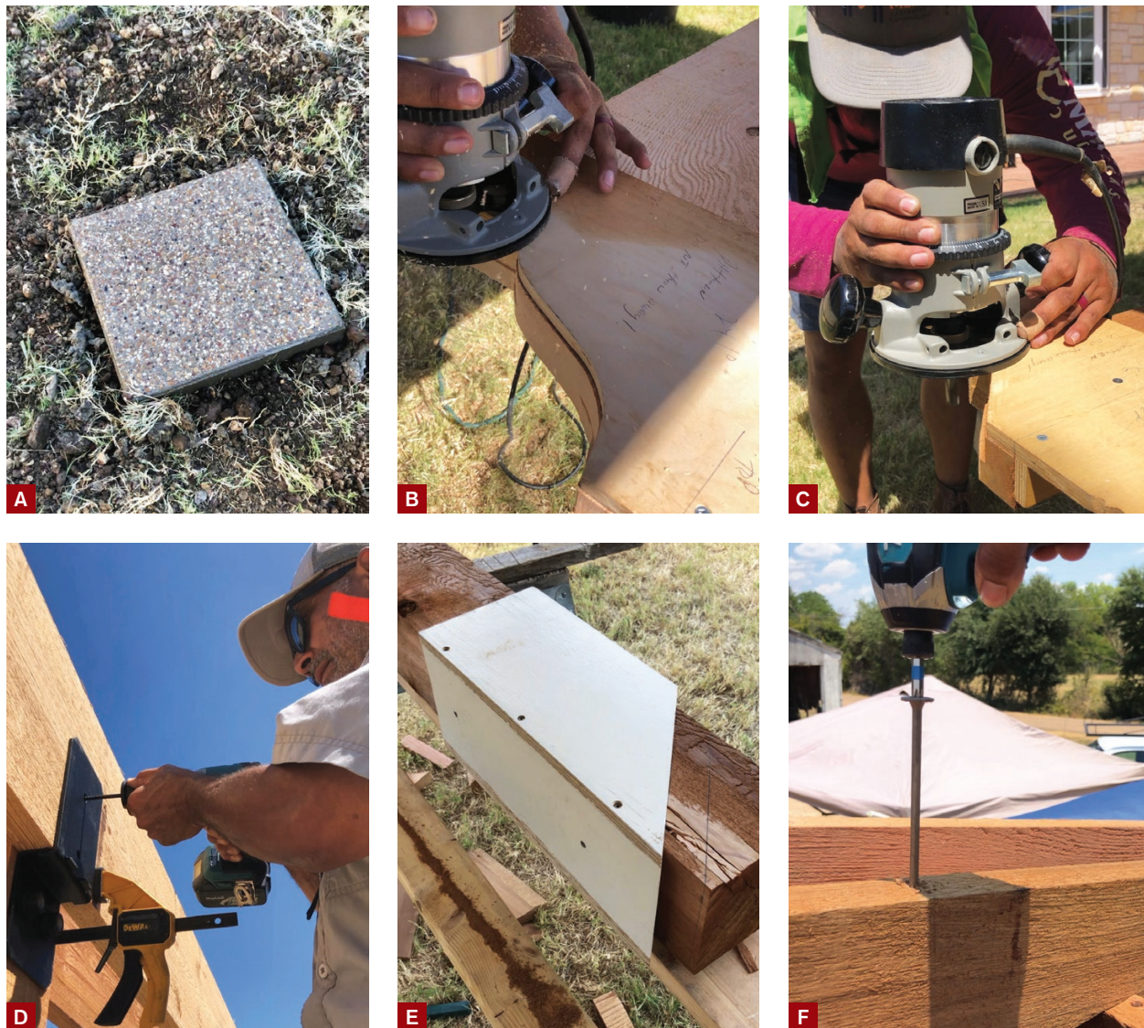
Figure 1. The pergola's support posts bear on the concrete patio and on 16-by-16-inch piers (A). The author uses one jig to shape the ends of the double 2x12 beams (B) and another one to shape the 2x6 rafters (C). Decorative hardware is used to hang the 2x12 beams from the pergola's 6x6 support posts (D). A simple guide made out of scrap material allows the author to make the clean and accurate 45-degree-angle cuts needed for the diagonal braces that reinforce the post-to-beam connection (E). Long structural screws fasten the 2x6 rafters to the beams (F).
