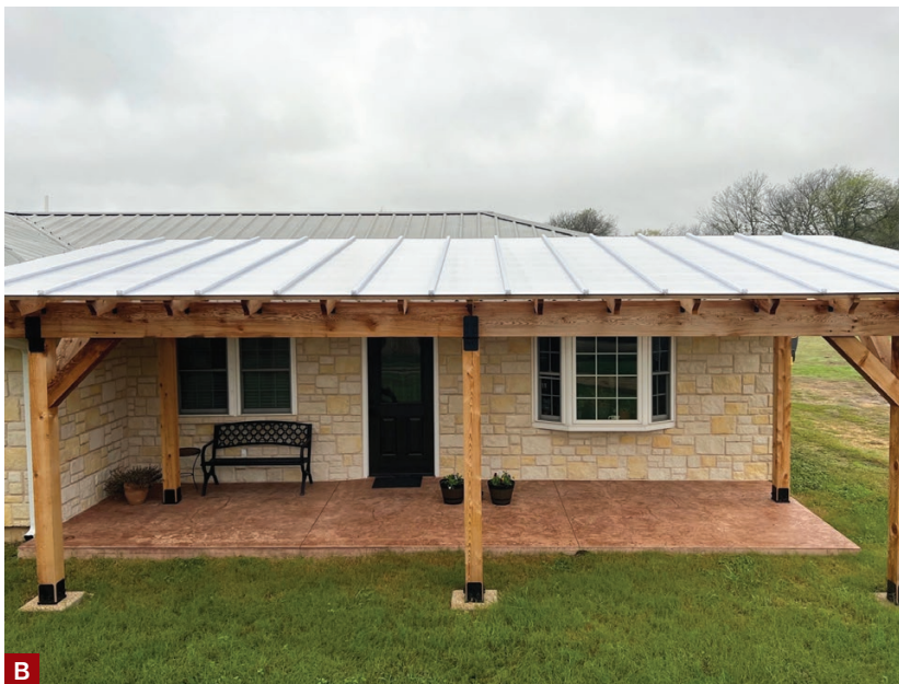
Figure 3. Raising the inner beam of the free-standing pergola above the eaves of the home's hipped roof allows for air circulation as well as the recommended slope (1 inch in 4 feet) for the polycarbonate roof panels (A). The panels chosen for this patio cover allow plenty of natural light into the home while providing shelter from rain and snow (B).
