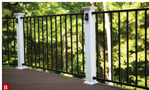
Figure 4. Another way the author streamlines the design and estimating process is by offering a limited number of railing options. Here, the same black aluminum railing panel is shown with two different post styles (A, B).
