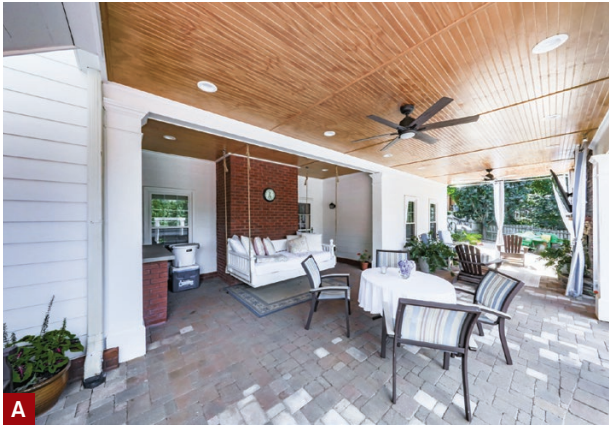
Figure 5. Under-deck ceiling options can also be standardized. The author's premium waterproofing package includes column wraps, wood ceiling, and crown molding (A). The basic package uses an aluminum under-deck system and costs considerably less.
