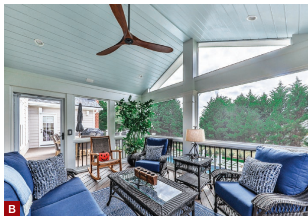
Figure 3. Two standard porch ceiling options offered by the author include exposed Douglas fir rafters and T&G roof decking (A) and standard roof framing with a T&G ceiling (B). Pricing for both is based on roof pitch and square footage.
