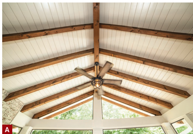
Figure 3. Two standard porch ceiling options offered by the author include exposed Douglas fir rafters and T&G roof decking (A) and standard roof framing with a T&G ceiling (B). Pricing for both is based on roof pitch and square footage.
