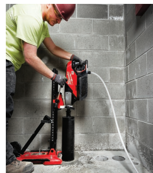
Milwaukee's MX Fuel core drill can be hand-held (left) or mounted in a drill stand for holes larger than 3 inches (right).
