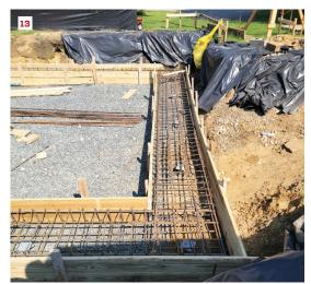
at the T-caps to reinforce the grade beam at the pier locations and about 12 inches apart between the piers. This cage was built on top of and centered over the pier T-caps and held off the stone by short lengths of rebar placed on top of the T-caps. This way, when we poured the concrete grade beam, the concrete would fill the gap between the stone and the rebar so that the steel would not be exposed.
