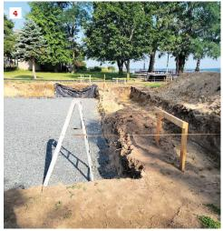
To account for the site's high water table, more than 7 feet of soil was excavated for the crawlspace foundation and replaced with a 3-foot layer of stone on top of filter fabric (1). To install the helical piers (2), the author uses a mini-excavator equipped with a torque head fitted with hydraulic pressure sensors that allow him to monitor the pier's installed torque (3). Batterboard lines were used to lay out the grade beam and pier locations (4).
