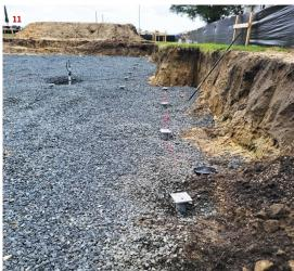
The torque, depth, and installation time and date of each helical pier were recorded on its T-cap and documented photographically (10). A total of 59 helical pierseach with a minimum bearing capacity of 15,000 pounds-were installed to support the grade beam footing (11).
