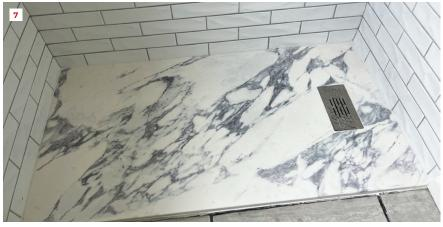
New floor sheathing and backerboard completes the rejuvenated shower area (4). The new cultured-stone base was first cut to fit the new space (5) with a hand-held tile saw equipped with a water spout, and then set in thinset. The base requires flanges provided by the manufacturer (shown along the end and back edge). These are secured to the edge of the base with screws before the wall tile is installed (6, 7).
