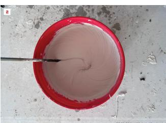
The author typically empties a box of joint compound into a 5-gallon bucket. Out of the box, the material is dry and stiff (1), but after mixing in about 1/2 cup of water (2), she gets a nice, smooth consistency that is vastly easier to work with.
