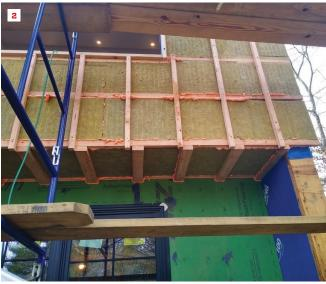
The author generously dusted the compacted earth with diatomaceous earth to protect against insects, laid down a 10-mil vapor barrier, and topped it with 2-inch (R-8) Rockwool Comfortboard 110 (1). A woven vapor barrier (not shown) was installed over the Comfortboard. A grid of horizontal strapping followed by vertical strapping was filled with Comfortboard 80 (2). Canned foam was used to fill any small voids, reducing convection and slowing vapor movement within the assembly.
