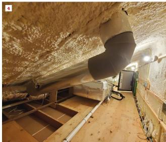
Walls shared with the garage received one thermal break with horizontal strapping and one layer of Rockwool Comfortboard 80 (3). In the attic above the mudroom and gym, the author created a 1-inch air gap below the roof sheathing with 1-inch XPS foam between the rafters, then applied 7 inches of closed-cell foam, for a combined R-value of around R-55 (4). The foam was carried down the walls to create a cohesive insulation barrier.
