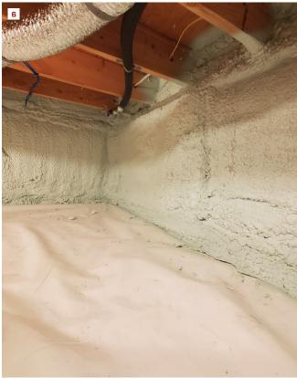
On the cathedral areas of the roof-ceiling assembly, the author added 2-inch strapping set perpendicular to the rafters and filled the voids with Rockwool 2-inch (R-8) Comfortboard 80 (5). In the crawlspace (6), one layer of 2-inch Comfortboard 80 was topped with CleanSpace, a 20-mil puncture-proof vapor barrier by Basement Systems. Closed-cell spray foam (R-16) locks the vapor barrier to the walls, connecting the wall insulation to the floor insulation.
