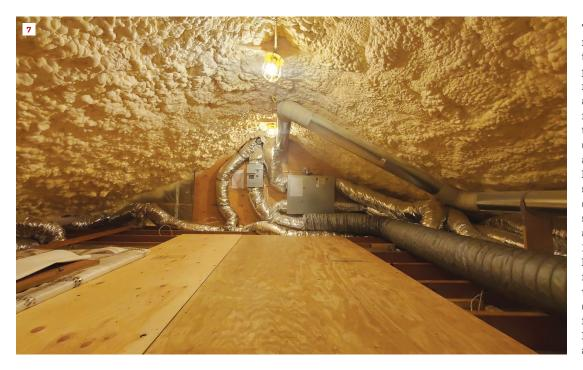
The author moved insulation to the roof plane, allowing mechanicals and ducting to remain inside the building envelope. First, a 1-inch air gap below the roof sheathing was created using strips of plywood as spacers and 1-inch XPS foam between the rafters topped with 12 inches of open-cell foam, for a combined R-value of around R-50.
