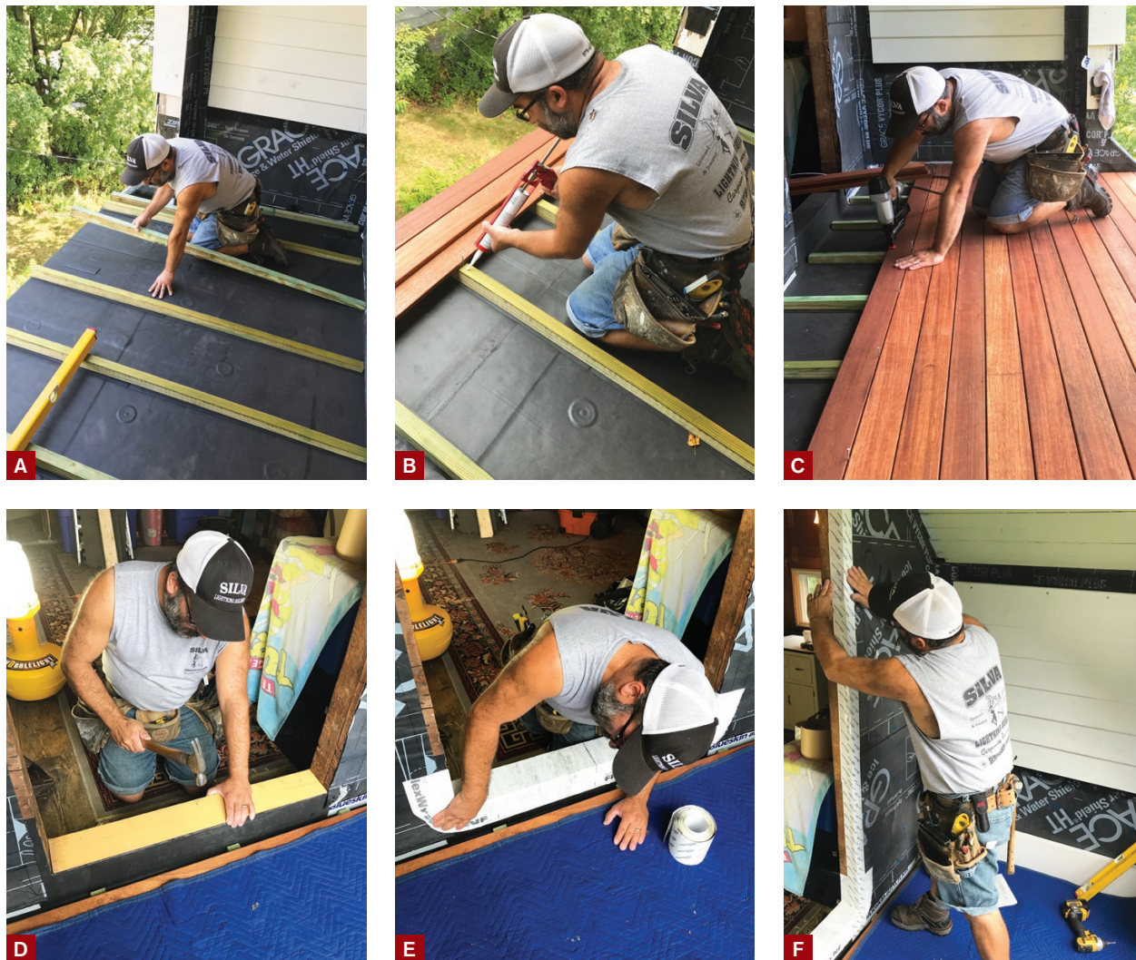
Figure 3. The author laid pressure-treated sleepers with a reverse taper over the membrane (A), then fastened 1x4 red meranti decking to the sleepers with marine-grade adhesive (B) and stainless steel nails (C). At the entryway to the attic, a short length of beveled siding tacked to the door sill over the membrane creates pitch for drainage (D). The author then waterproofed the sill with flexible flashing tape, which wraps up the jambs (E), then used regular peel-and-stick flashing tape to seal the sides of the opening to the WRB covering the wall (F).
