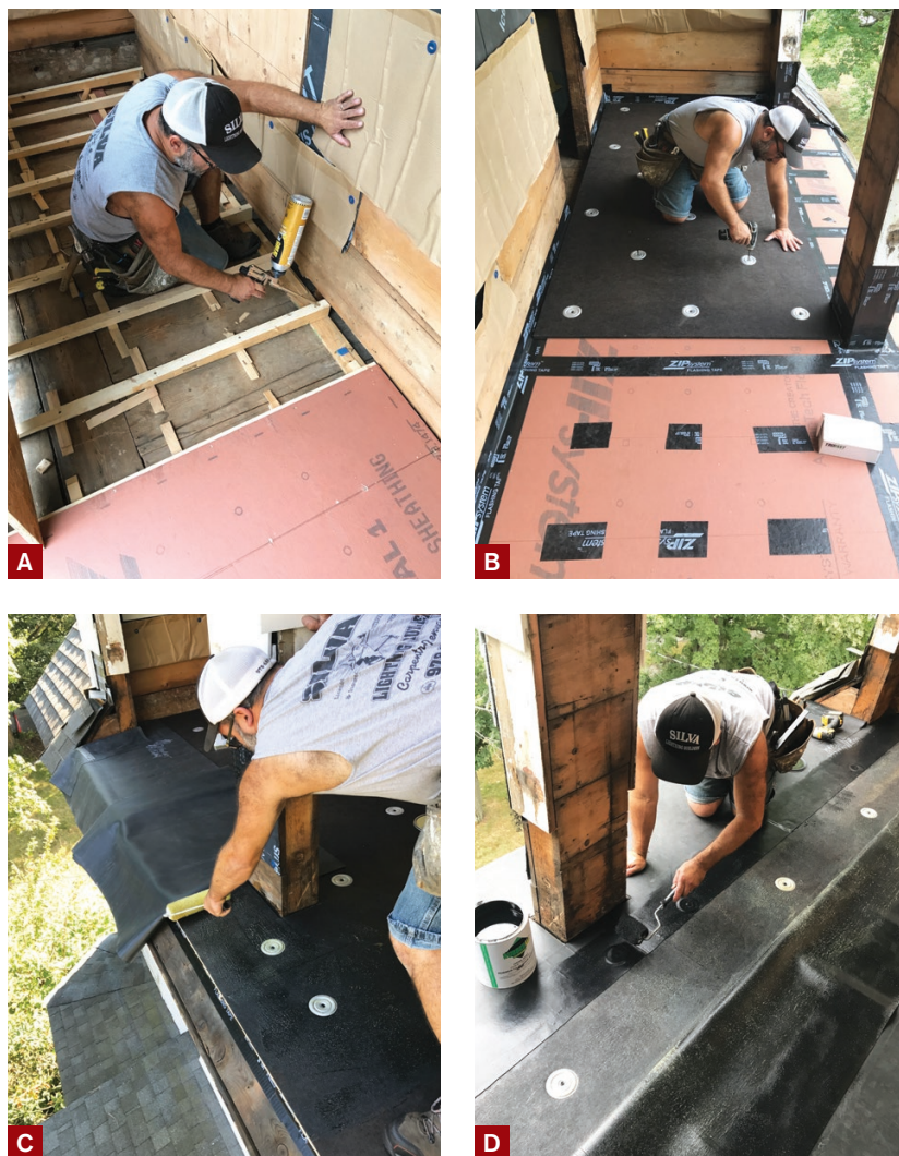
Figure 1. The author installed tapered sleepers followed by Zip sheathing to pitch the roof deck away from the house (A). Then he installed recovery board over the sheathing (B), followed by the EPDM roof membrane (C). The author used a neoprene bonding adhesive to glue the membrane to the underlayment, and a rubber-to-rubber adhesive at lap joints in the membrane (D).
