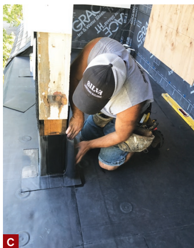
Figure 2. The author flashed the column with four pieces of membrane folded and cut to fit, starting with the outside face followed by the two sides (A). Rubber-to-rubber adhesive was used to adhere the legs of the last section of membrane on the inner face of the column to the previously installed pieces (B, C). At the sides of the balcony, the author used butyl-based flashing tape to isolate the EPDM roof membrane from the asphalt-based Vycor flashing (D).
