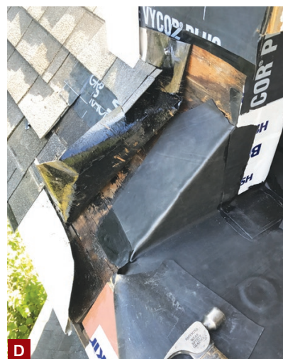
Figure 2. The author flashed the column with four pieces of membrane folded and cut to fit, starting with the outside face followed by the two sides (A). Rubber-to-rubber adhesive was used to adhere the legs of the last section of membrane on the inner face of the column to the previously installed pieces (B, C). At the sides of the balcony, the author used butyl-based flashing tape to isolate the EPDM roof membrane from the asphalt-based Vycor flashing (D).
