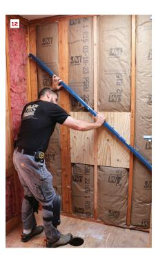
The author checks for plane by spanning a 6-foot-long level across an existing studwall, revealing a gap between a stud and the level (9); the stud will be shimmed later. Here, a stud crowned outward is power-planed (10). The author rechecks the wall for plane after installing grab-bar blocking (11, 12). Note: The unfaced batts are in a party wall between town-house units.
