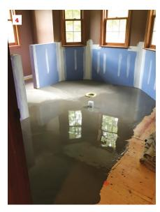
Floor systems need to be strong and stiff enough to support tile, but often in an existing home, they are underdesigned, out-of-level, and structurally compromised (as shown here) and need to be evaluated by a design professional (1). When pouring liquid-applied self-leveling compound, the author first sets screws to a level elevation using a laser, paints the screws fluorescent orange to stand out (2), then works the compound flush to the tops of the screws (3), feathering it out to level (4).
