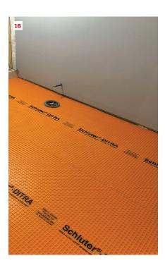
To help with jobsite communication, the design plans are posted on the walls, and the locations of critical items are marked on blocking and studs (13). On a wet wall, a metal protection plate (below the controls) was recessed flush with the face of the framing (14). The floor surface is vacuumed (15), then the uncoupling membrane is thinset to the underlayment (16).
