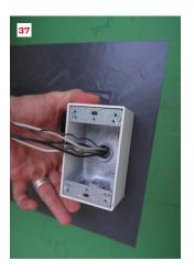
**Penetrations.** For any penetration through the exterior, the author's goal is to limit its size. When the author was off site, electricians installed the wrong type of exterior outlet (35). The author corrected this by removing the box, patching in the sheathing (36) and using a surface-mounted metal box so only the wire, not the entire box, needed to be sealed (37).
