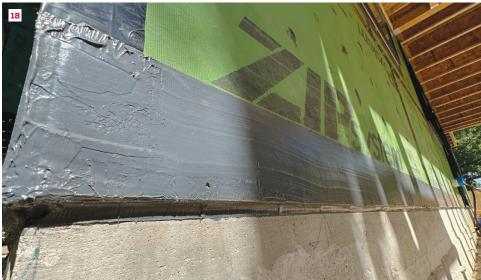
Foundation-to-wall seal. At the base of the wall, the author's crew uses painter's tape to establish a clean line at the top and the bottom (17). The tape makes it look nice, but it also allows the installer to apply a thick bed of sealant that is free of pinholes—a detail that trying to feather the edge to a chalk line won't effectively achieve (18).
