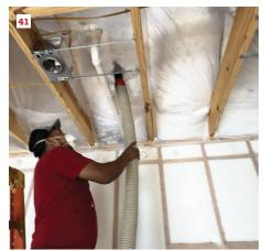
Thermal control is achieved using 1-inch (R-3) Zip-R sheathing on the walls (38) and roof (39) to limit thermal bridging. (Note: In colder climates, thicker foam would be needed for continuous insulation.) The author fills the cavities with blown-in fiberglass (40). In attic areas, he drapes the netting to create a "bag" that can be filled with more insulation than the depth of the framing would otherwise allow (41).
