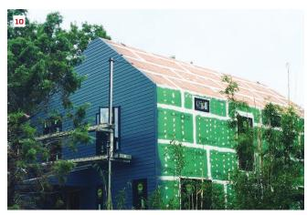
**Block and caulk.** On a new build, the author used DuPont's fluid-applied barrier in concert with Zip System sheathing (6-8). Zip System was new to the author at the time, and he had more confidence in "finger painting" with fluid-applied than sealing panel seams with tape. It was on this and another, simultaneous new home that "block and caulk" was born (9, 10).
