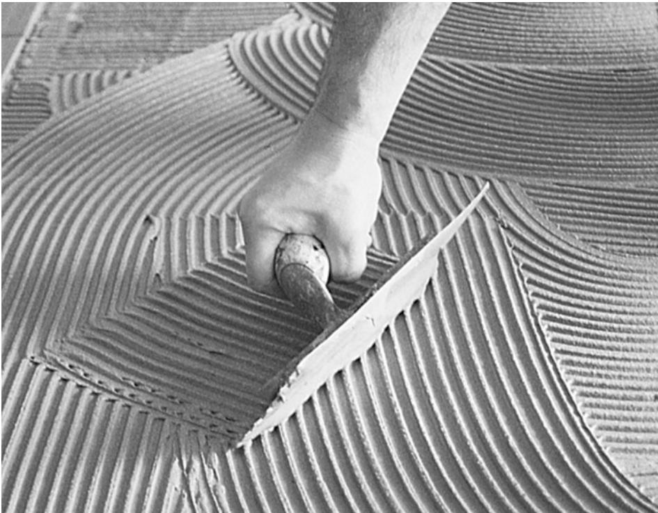
FIGURE G: APPLYING TILE ADHESIVE
